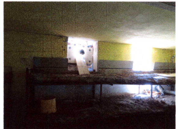
IMAGINE INTERIOR SUBSOL
